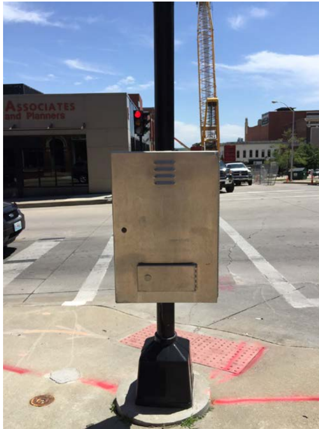
Front View (South)
