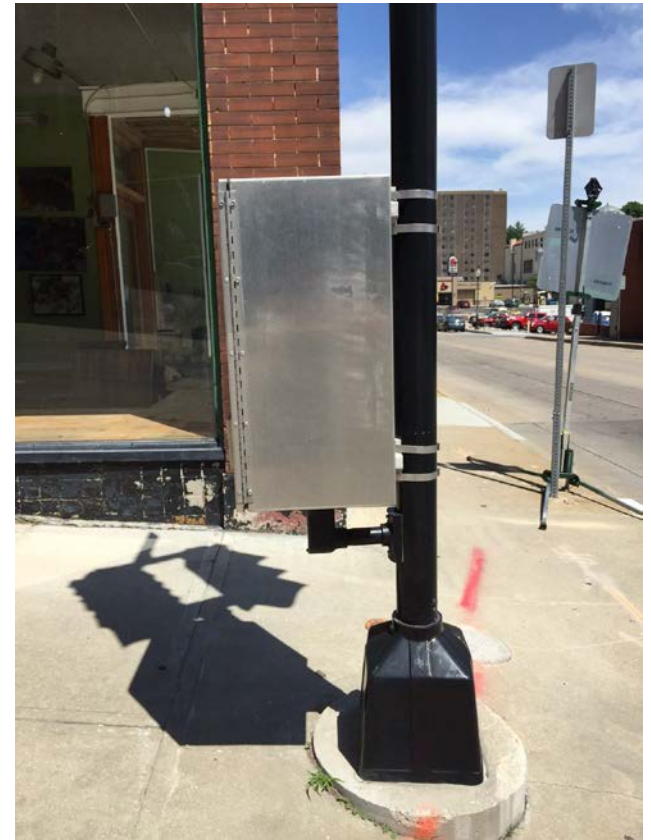
Side View (East)
